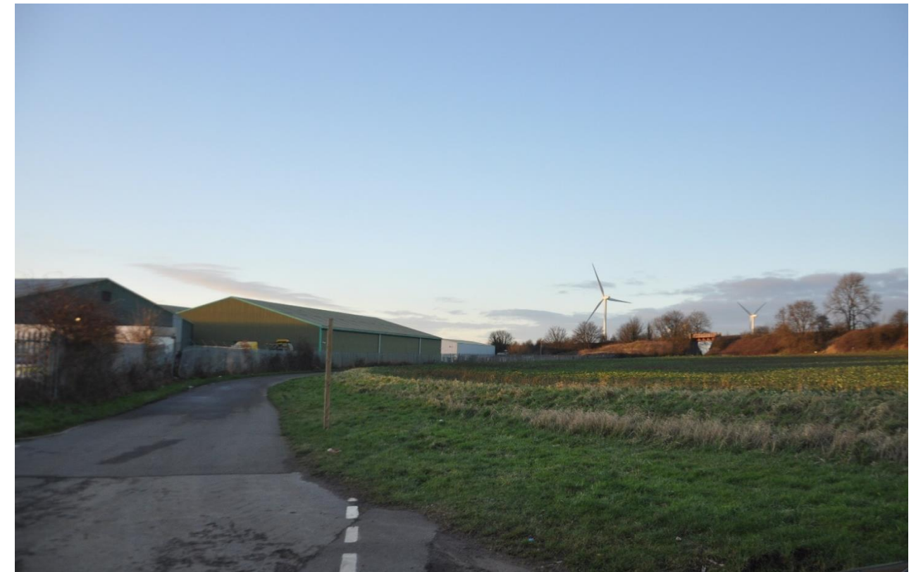
Figure 2-29 View 2.5, Northwest – Access road leading to private property. Unilluminated.
