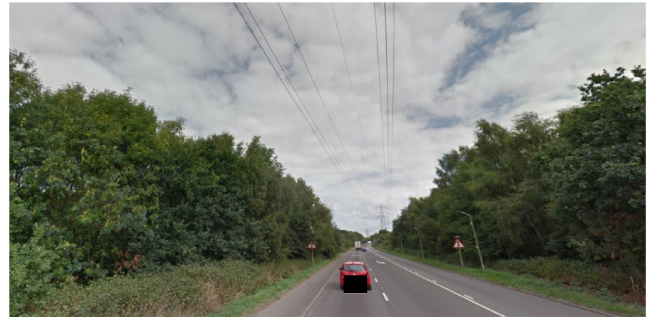
Figure 2-45 View 3.4 East – South – Phoenix Parkway (A1077).
