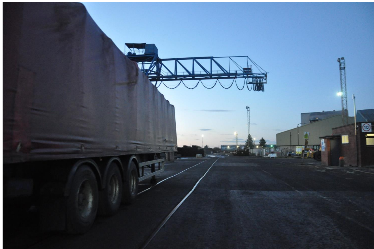
Figure 2-16 View 1.3, North - Flixborough Industrial Estate.
