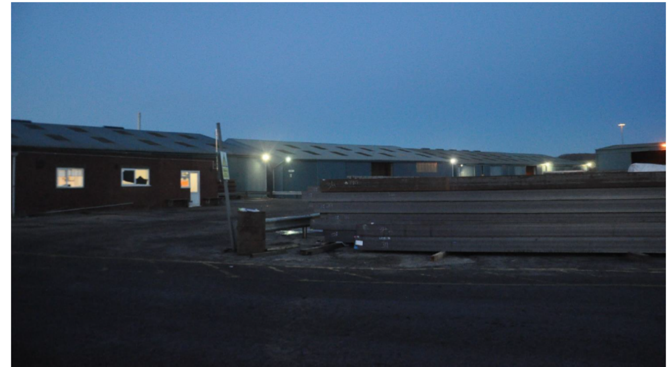
Figure 2-10 View 1.3, East - Flixborough Industrial Estate Storage area.
